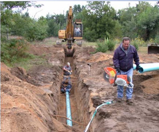
Sewer main installation gets underway
