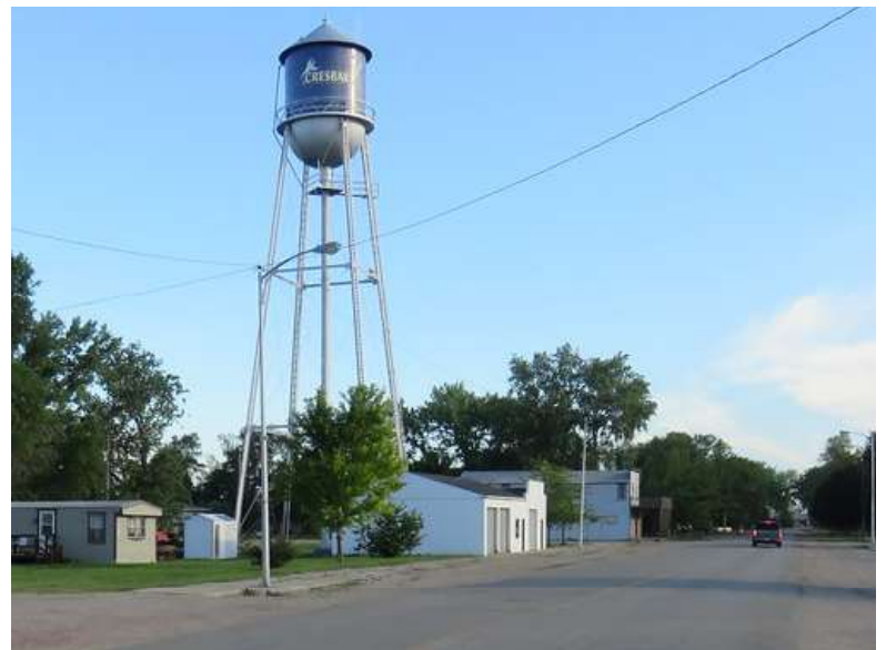
Above: City water tower and street
